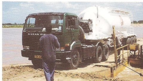
Supplying cement by tanker to Rufiji bridge project.
